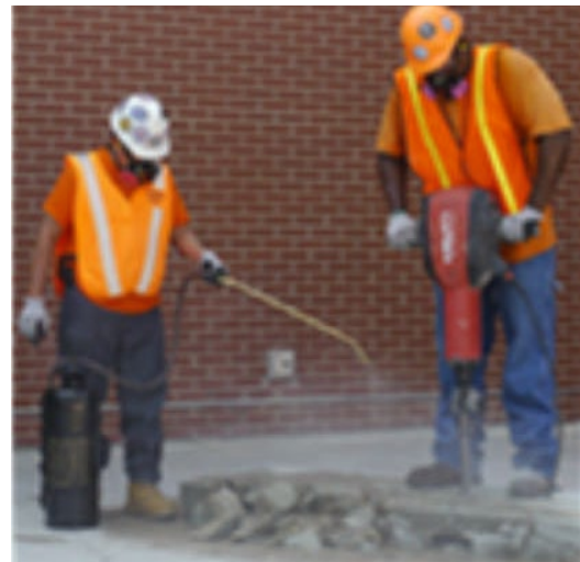
One worker applies water using a portable sprayer to suppress dust while the other jackhammers.
