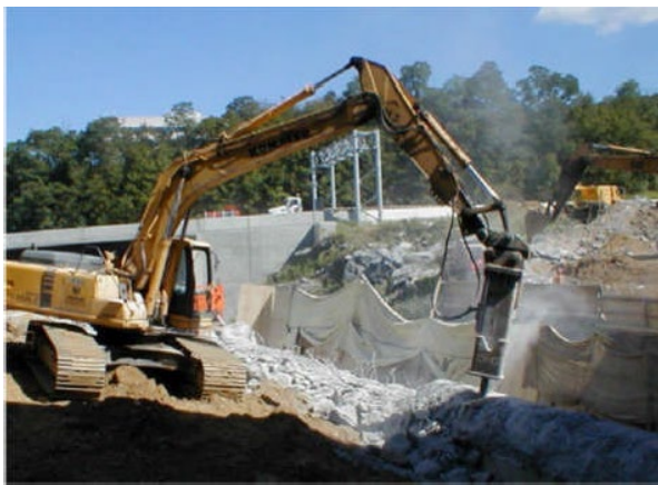
Excavator equipped with an enclosed cab and hoe-ram demolishing a concrete wall.
